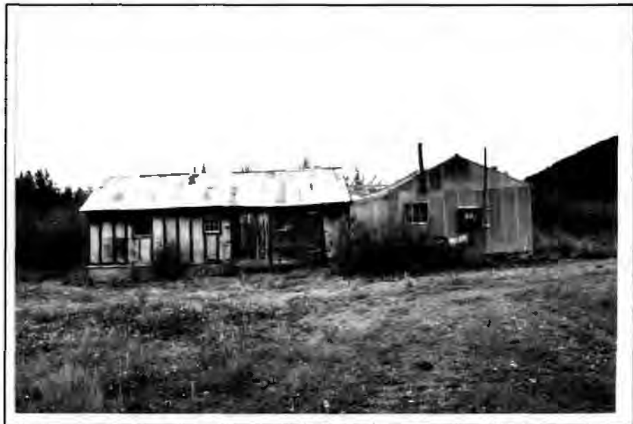
Figure 154. The Workshop and Garage, 1993. The view is looking west.
